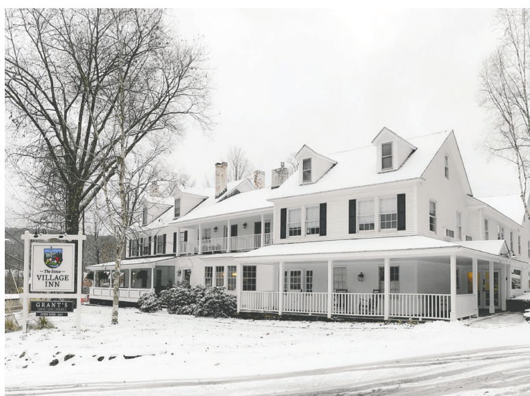
The historic Stowe Village Inn is home to Grant's Bar & Restaurant, elegant interiors, and rooms in the Main Inn and Modern Motel.
